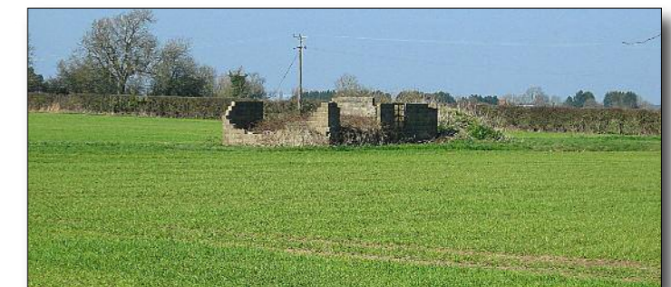
Remaining evidence of Market Garden on Horsegate Field Road, breeze block packing shed built by Roger Hepworth. Photograph Elizabeth Fincham.
