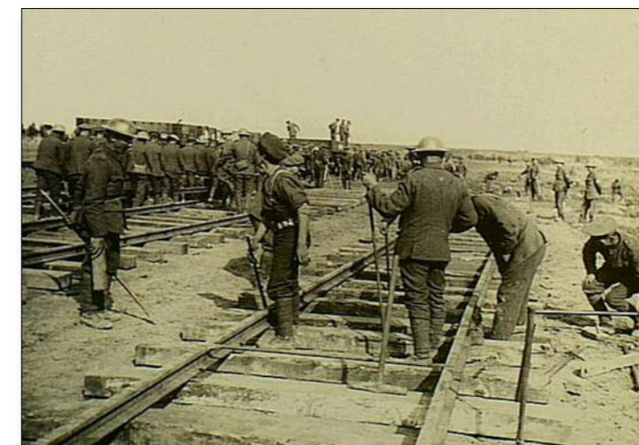
British army engineers constructing new railways in France. A role carried out by Charles Lamming and Fred Rusling. Copyright Australia War Memorial
