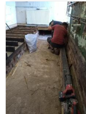
Half way through removing the rotten timbers.
